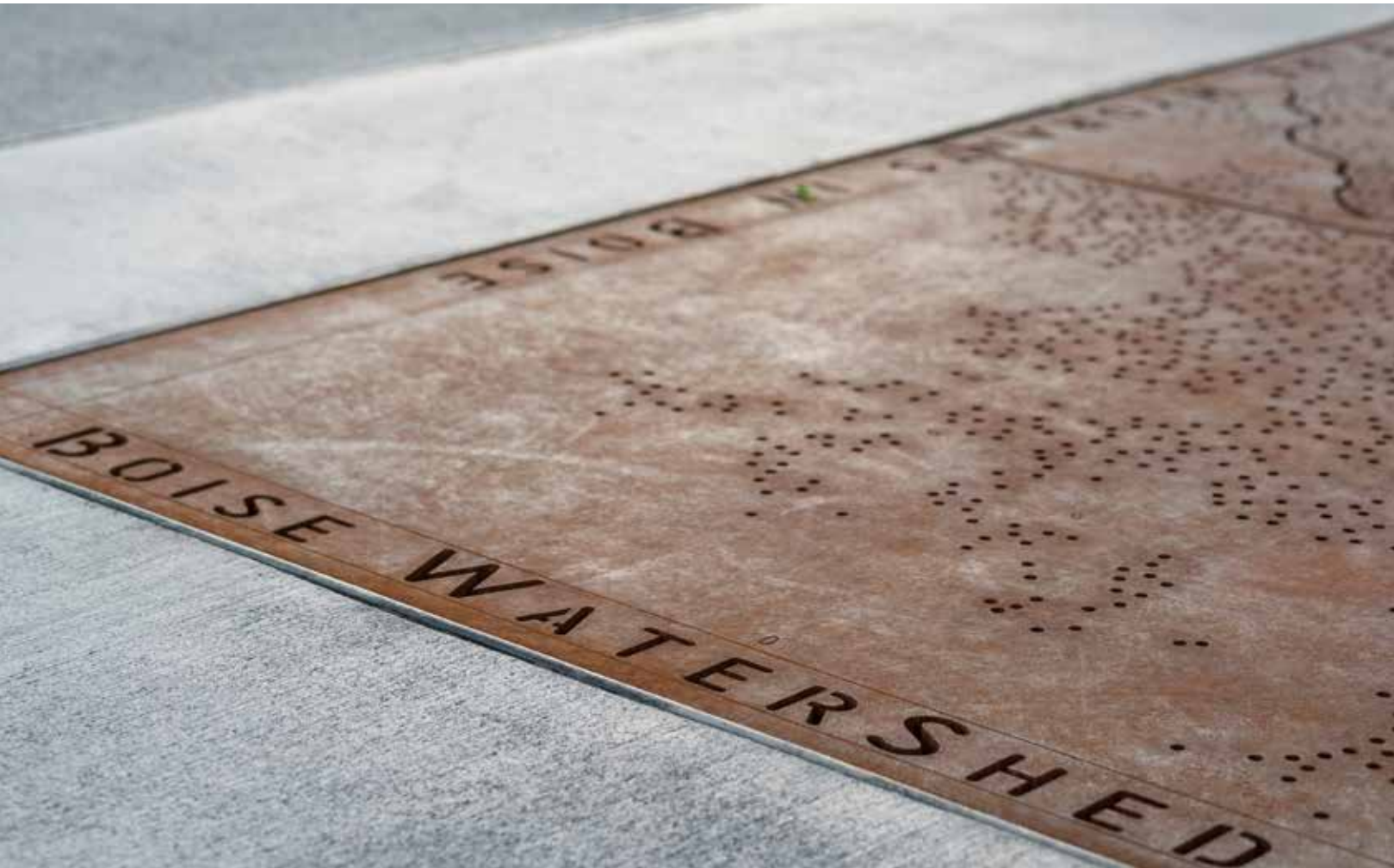
Using infrastructure maps, Amy Westover created three different tree grate designs for Boise WaterShed's River Campus. Mapping Infrastructure detail (2016) by Amy Westover, photo courtesy of Arts & History
