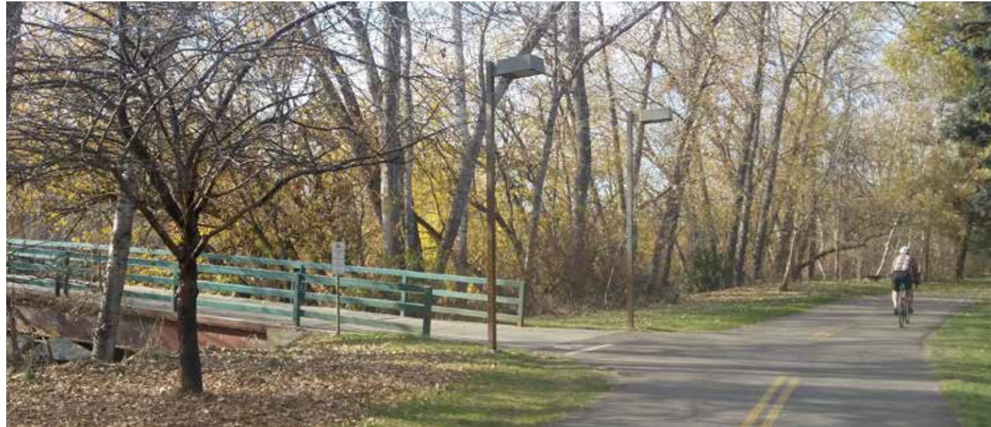
Existing street lights, like this one near the Green Belt, could be augmented or replaced with solar street lights, photo courtesy of Arts & History
