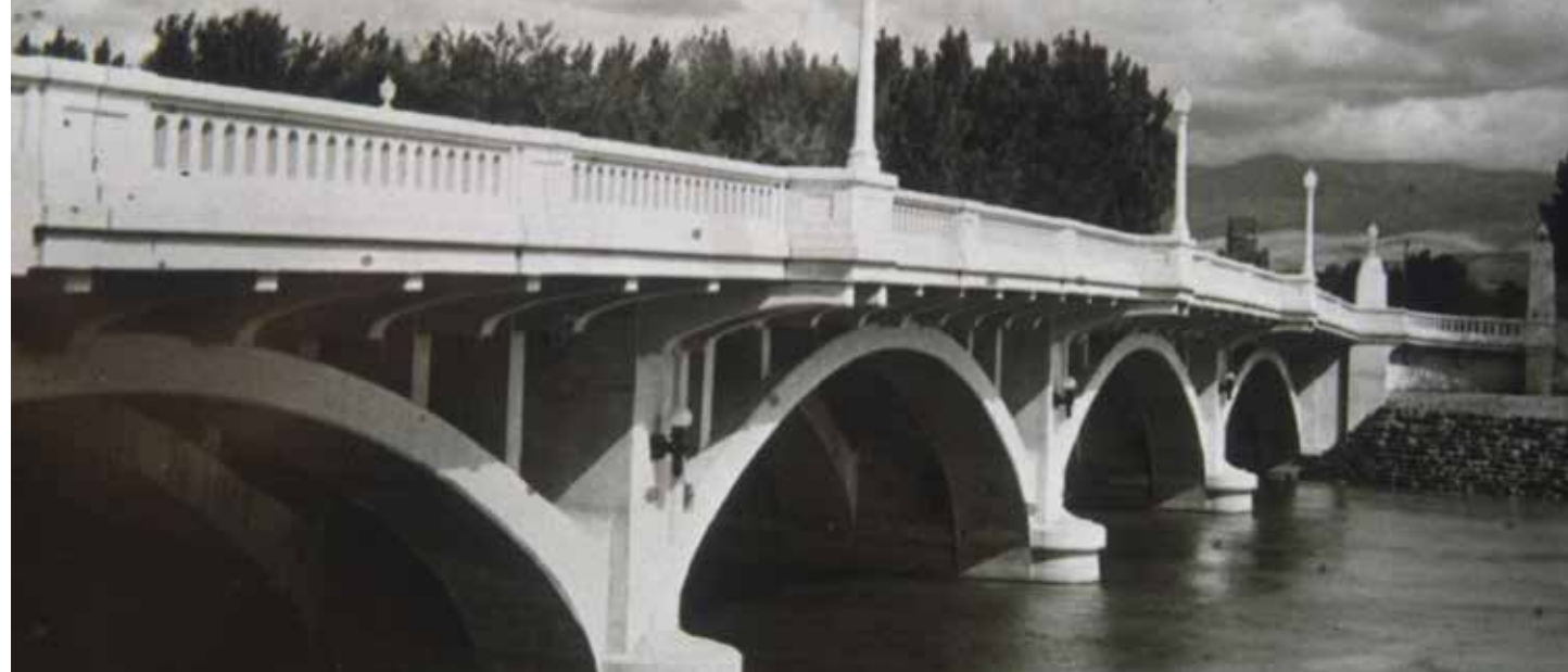
Oregon Trail Memorial Bridge, photo courtesy of Boise City Archives
