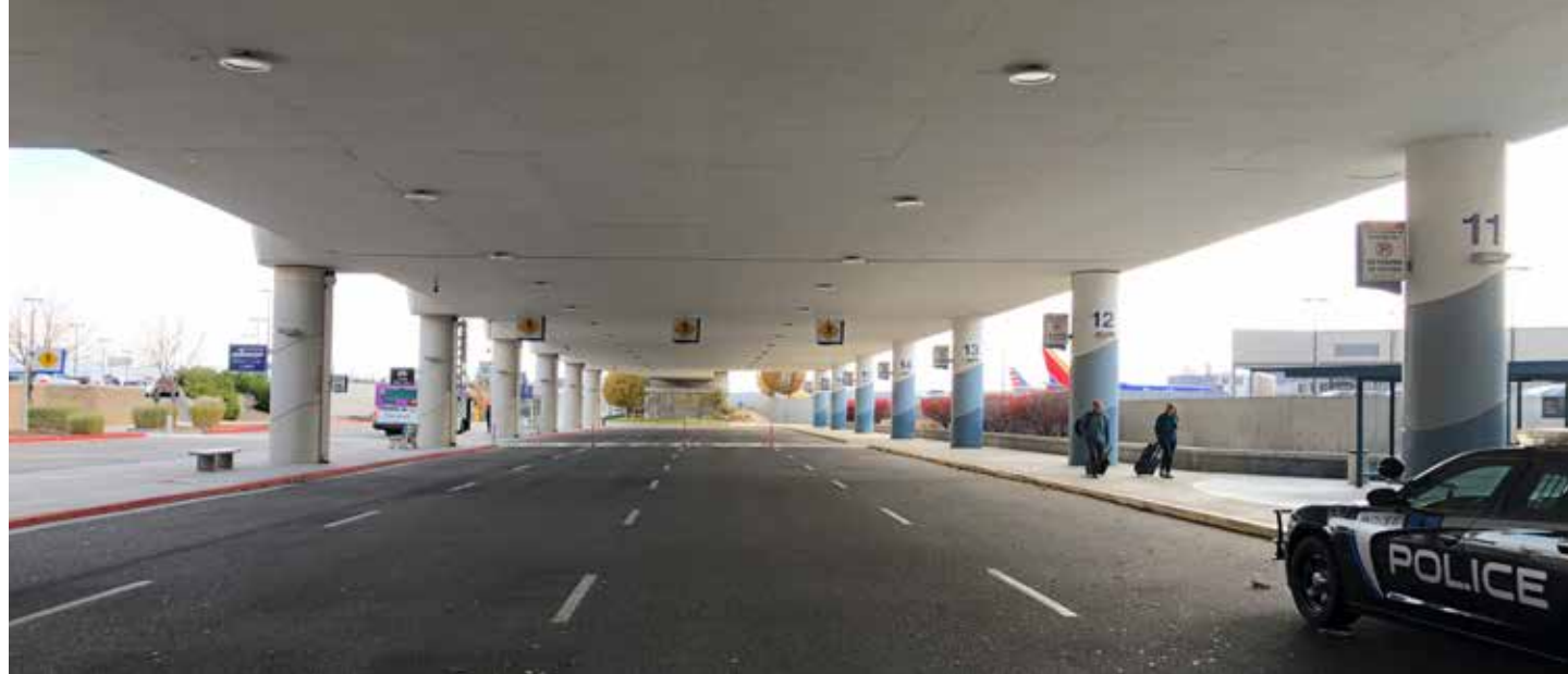
Boise Airport lower roadway ceiling, photo courtesy of Arts & History
