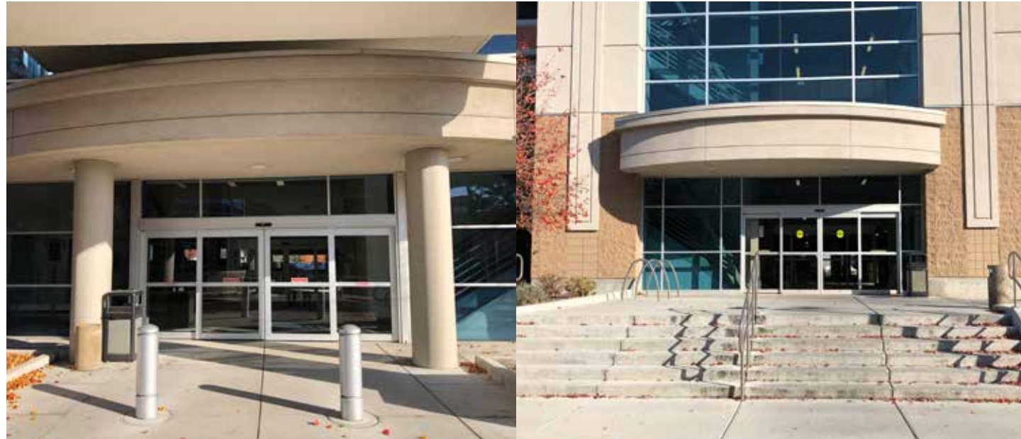
Exterior entrances to Boise Airport parking garages, photo courtesy of Arts & History
