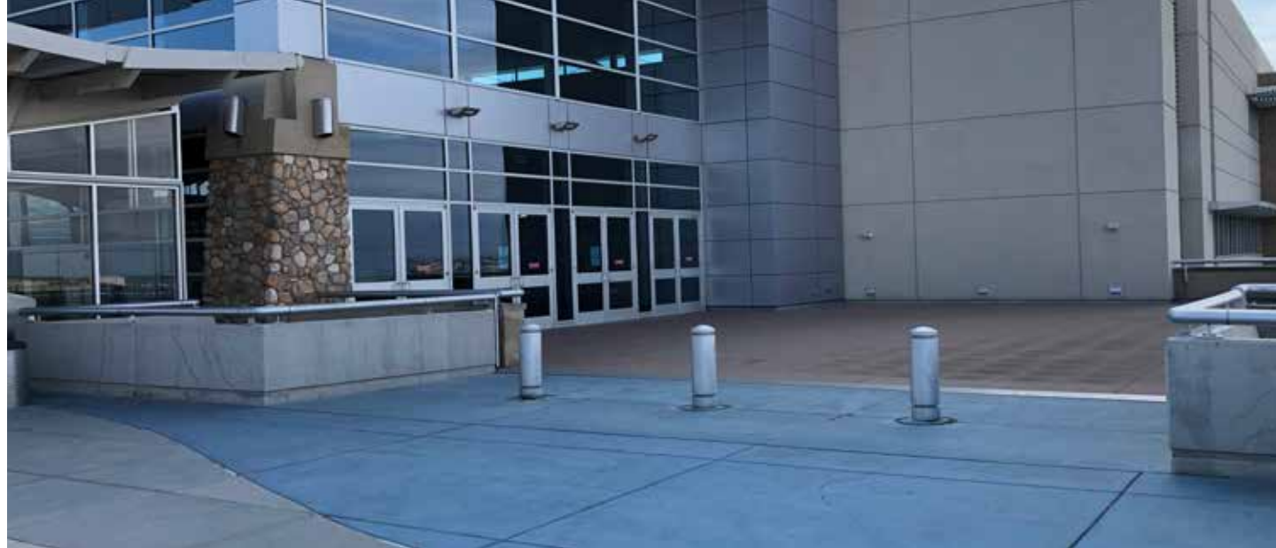
Boise Airport upper roadway entrance plaza, photo courtesy of Arts & History
