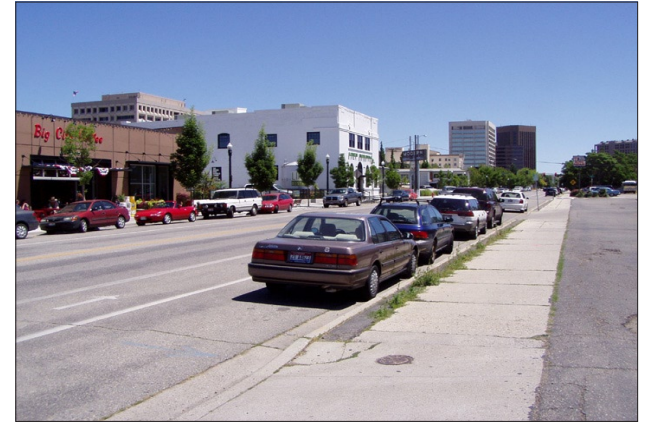
View of an unimproved edge of Grove Street.
