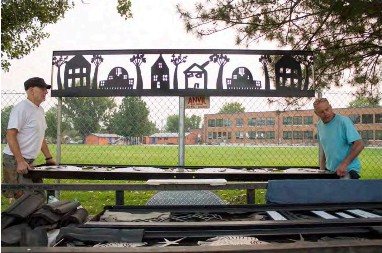
Michael Cordell and Dennis Proksa installing Whittier Fence art project on Whitewater Boulevard.
