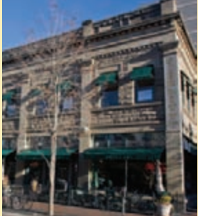
The Fidelity Building, 1908 A.F. Montandon advertised this Romanesque, multi-use structure as “the most up-to-date business block in Boise.” The building earned its current name after Fidelity Adjustments took the 2nd floor in 1922.
