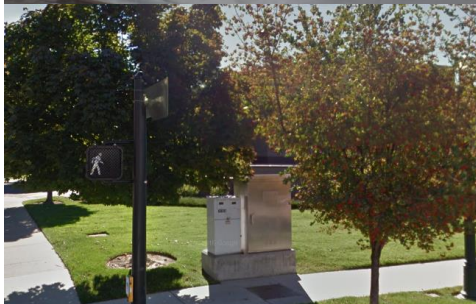
2 nd & Front, SE Corner
