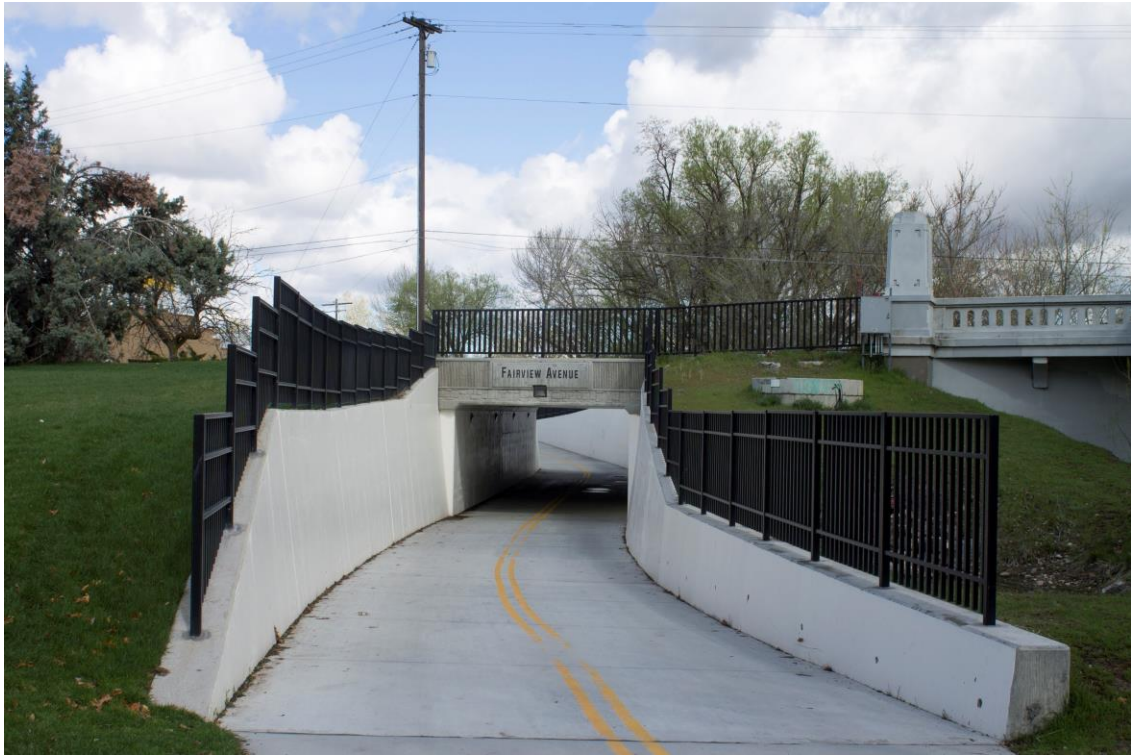
Site View Looking West
