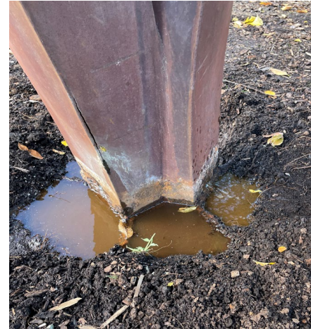
Figure 4: Observed corrosion at "History in Motion" by Mark Stasz
