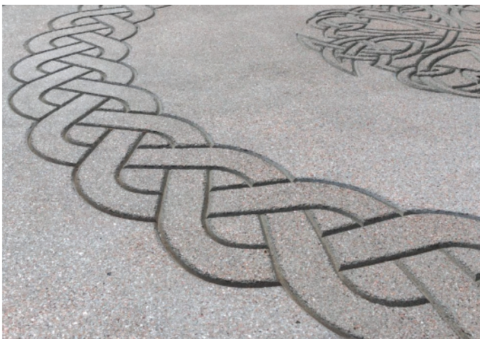
Storylines - stamped concrete PMC 780 Urethane Rubber 1/8"
