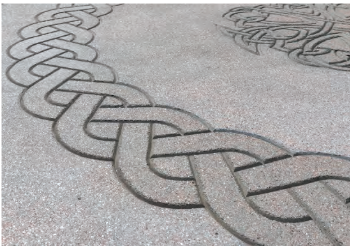
Storylines - stamped concrete PMC 780 Urethane Rubber 1/8"
